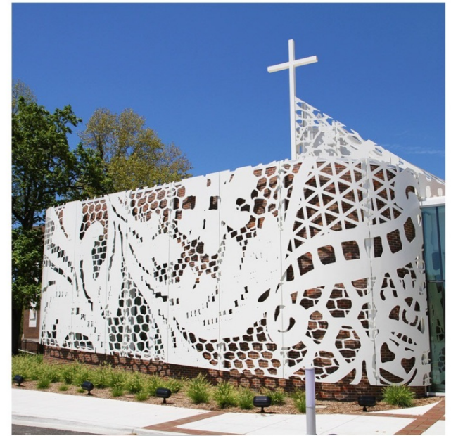
DESIGN REALIZED AFTER A THREE DAY INSTALLATION SET THE FORTY-FOUR PANELS IN PLACE
