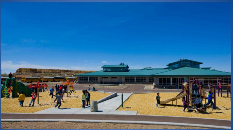
The design achieved a 30% energy savings over similar sized schools. There is a system to capture and save rain water that flows off the metal roof and is then used to supplement the landscape irrigation system. The building orientation and roof overhangs provide passive shading to help keep the building cool during the days of intense sun.
