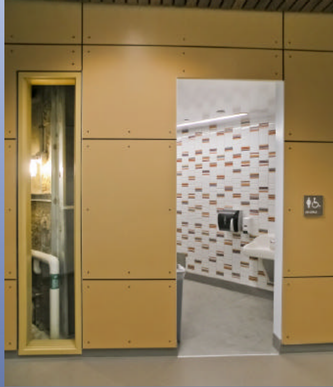
"Truth" wall: Building systems are exposed from the main hallway.
