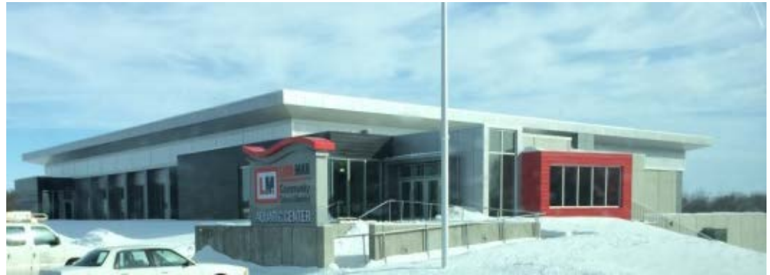
Existing Aquatic Center
