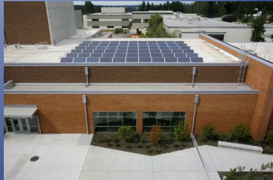
Photovoltaic array visible from stairwell in adjacent wing (the original building can be seen in the background, before demolition)
